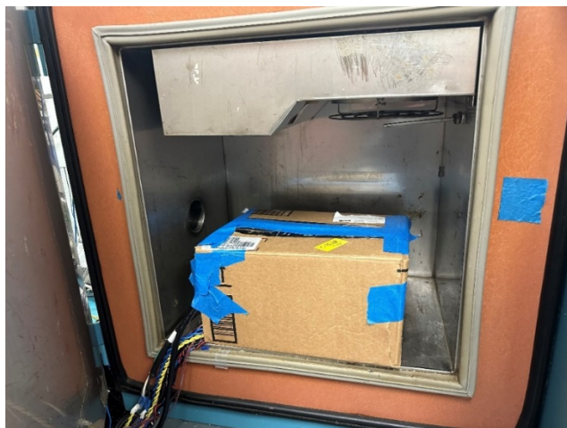
Figure 68 – Unit Placed Inside a Box to Prevent Air Flow.
